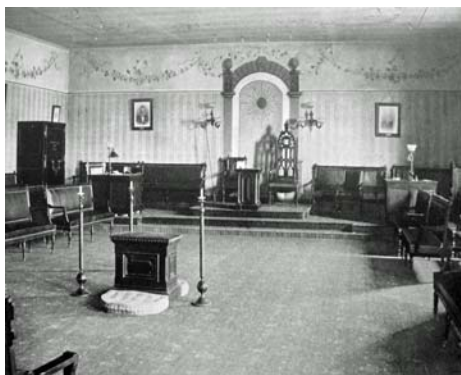
Old Lodge Room – East View
